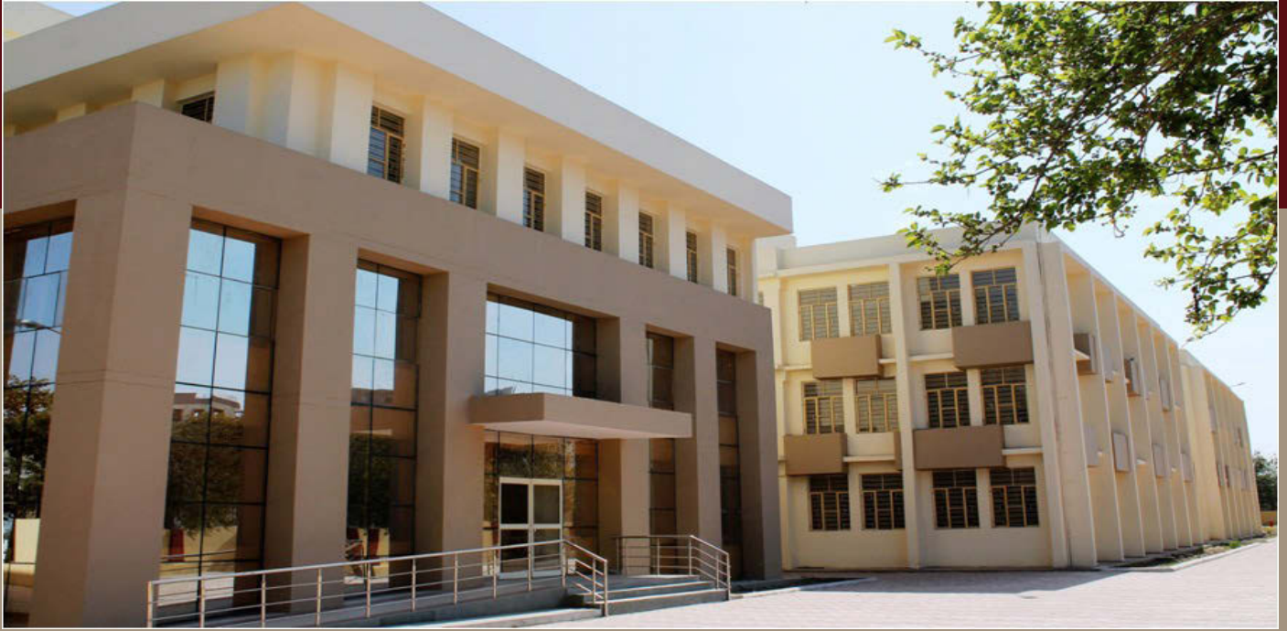
Newly constructed building of Kendriya Vidyalaya sector-25 Rohini, New Delhi
